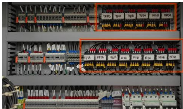
Gambar 4.4 Rangkaian Hardware Trip Multi Feeder
